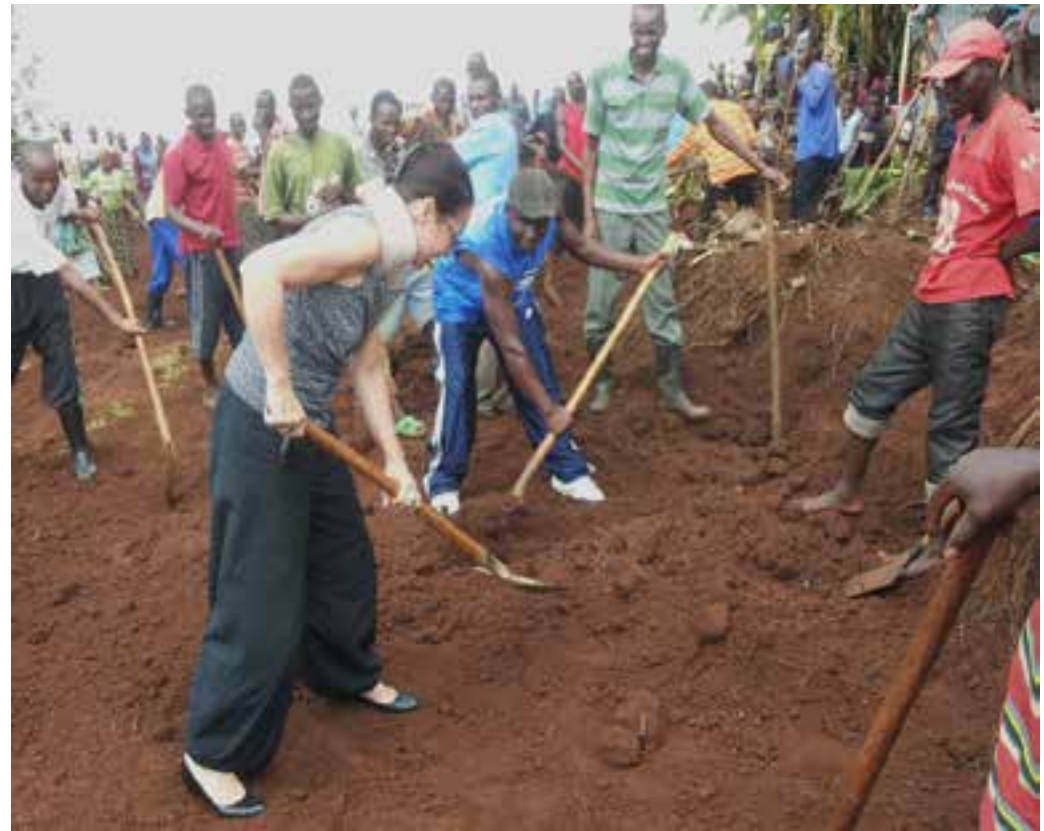
building the new roads for «Rudakabukirwa», Gasabo District
