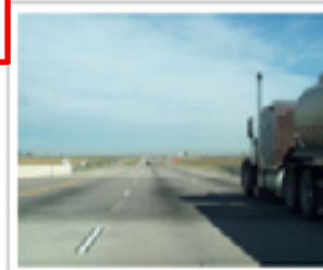
An Interstate Highway bridge with an asphalt overlay
