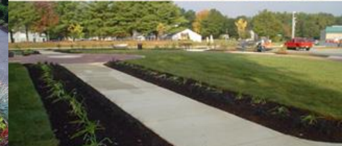
Completed Water Quality Park with Underground Terre Arch Stormwater Retention System
