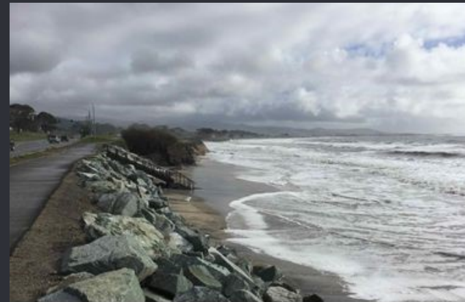
Erosion and coastal squeeze Surfer's Beach, San Mateo County January 2017
