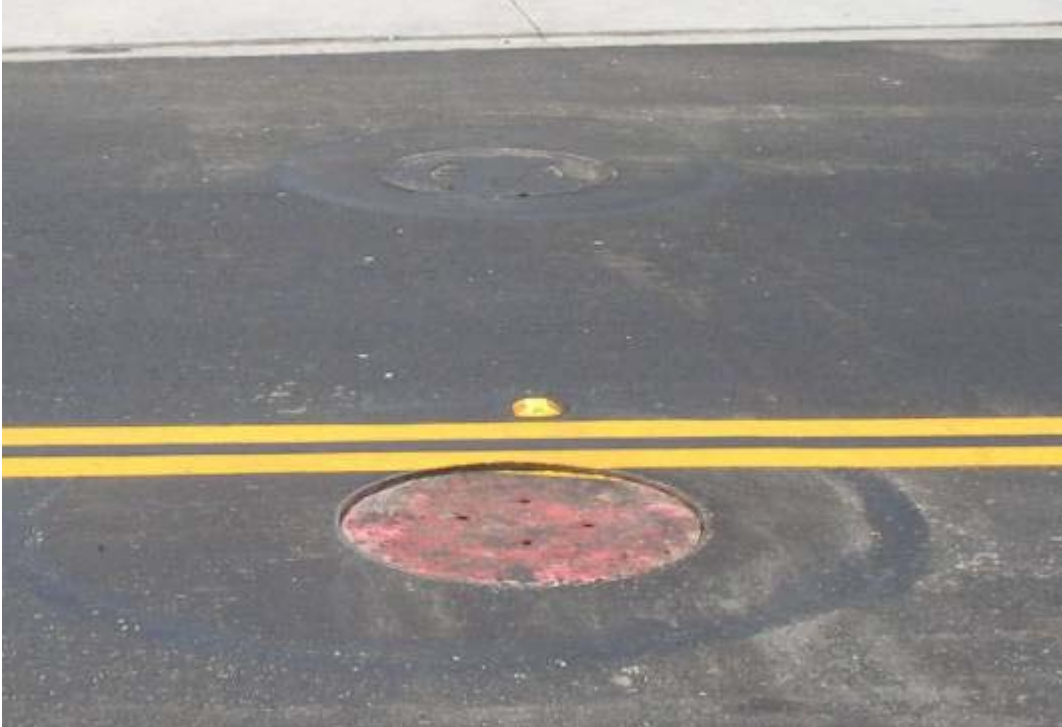
Figure 5 – Street-overlay complete (OCSD new frame and cover shown at top)
