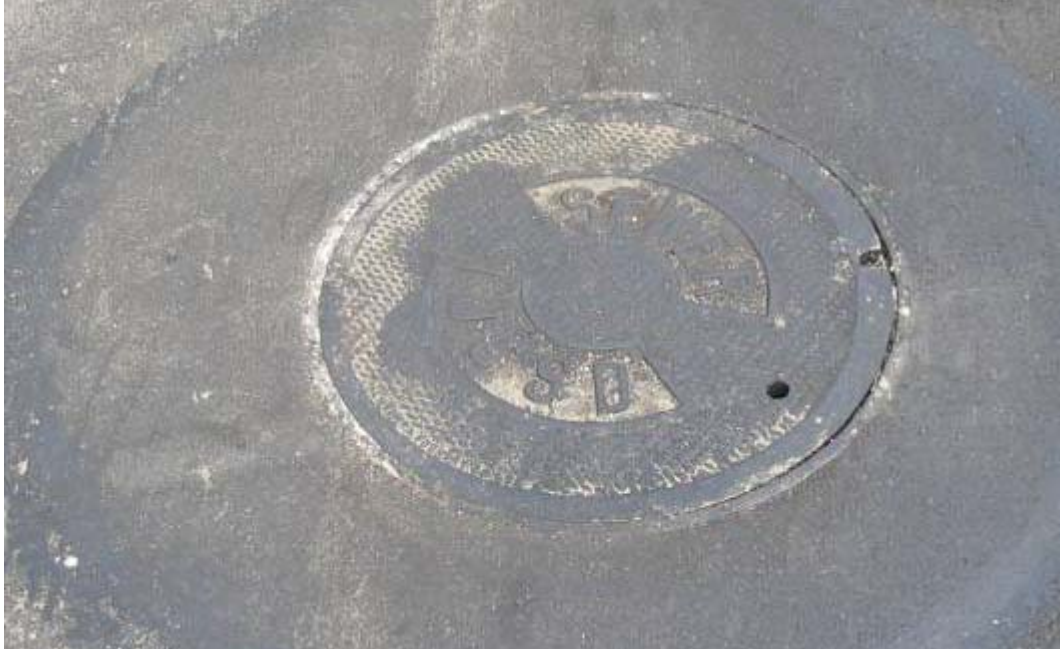
Figure 7 – New OCSD frame and cover after street-overlay is complete
