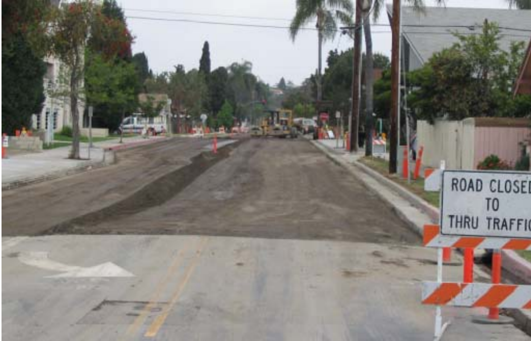
Figure 2 – Street Overlay in progress along Highland Ave.
