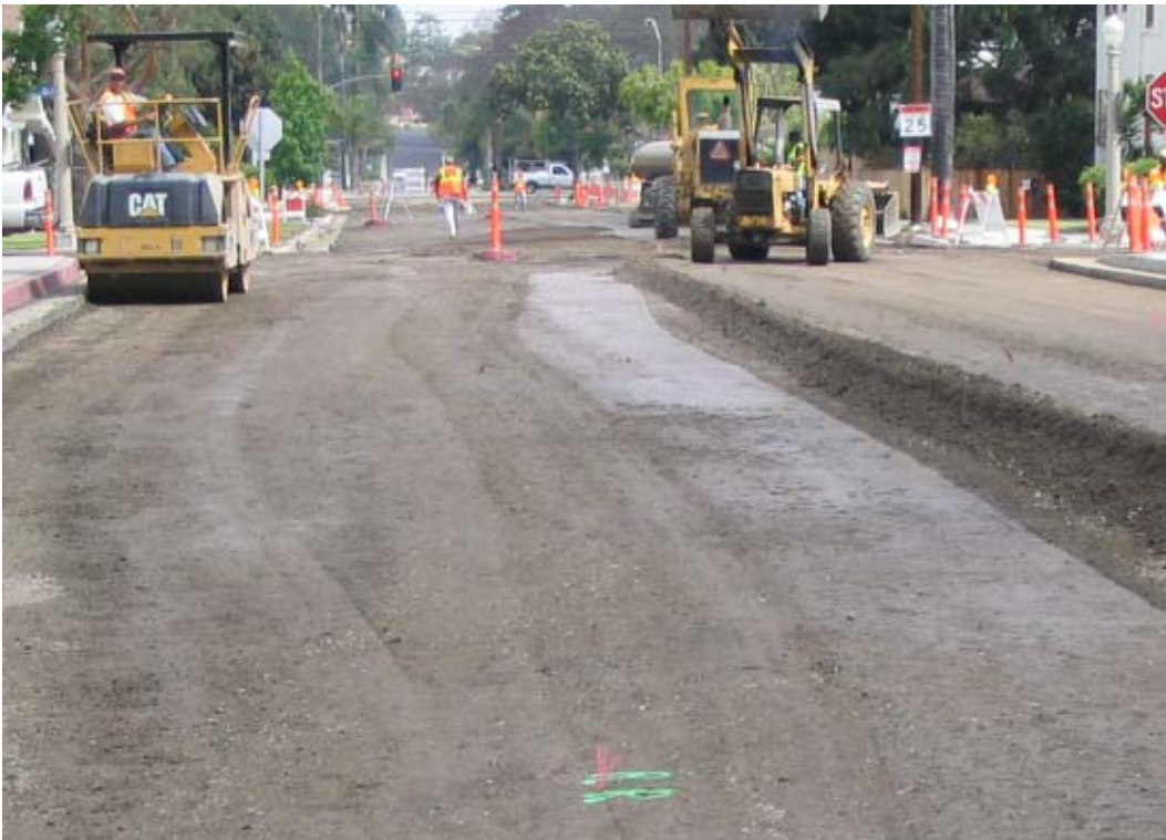
Figure 3 – Buried steel plate marked by “RR”
