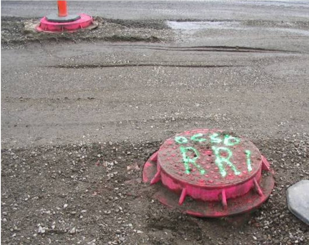
Figure 4 – Frames and covers ready to be removed (OCSD shown at bottom)
