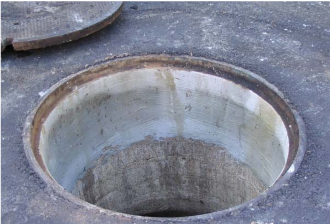
Figure 13 – Figure 12 manhole after contractor repair
