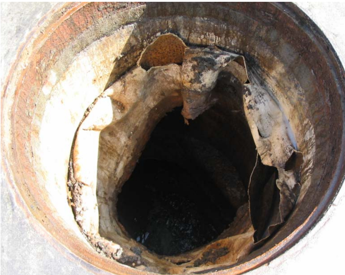
Figure 16 – Same manhole in Figure 15 after street-overlay work is complete
