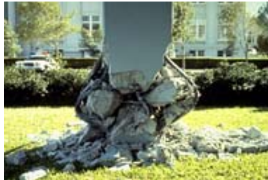
1979 – Imperial County Services Building
