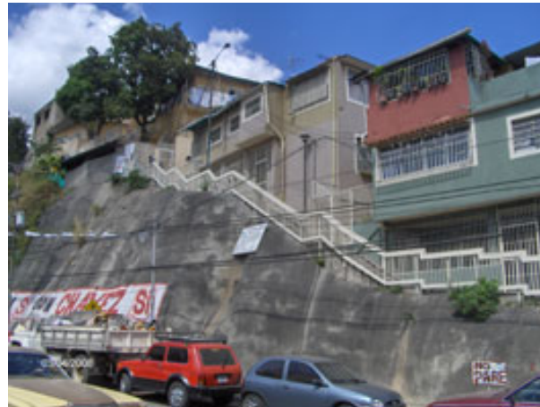
Graphic 14: Façade Improvement Project.
