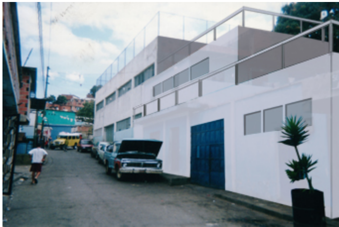
Graphic 9: Refurbished Community Building.
