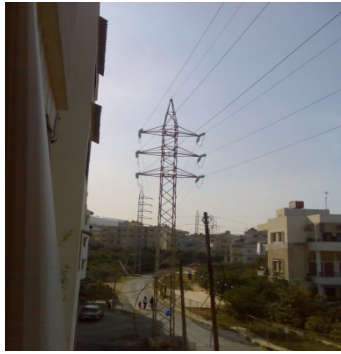
Fig.2: transmission lines near residential areas
