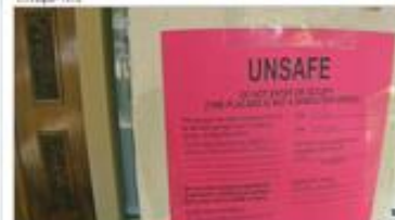
Image of a red-tagged building in Napa, Monday, Aug. 25, 2014.
