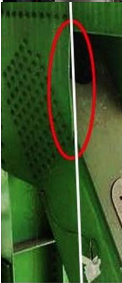
The ill-fated, warped U10 g bridge. June
