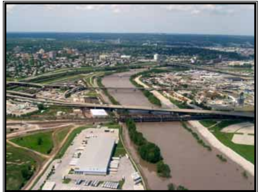
Photo from USACE, Kansas City District website
