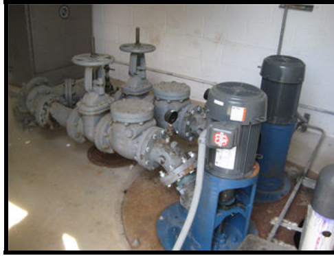
Figure 4. Wastewater pumps at MCAS Cherry Point
