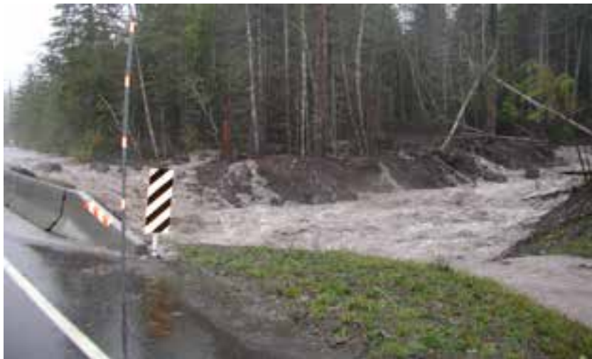
Properly sized drainage structures
