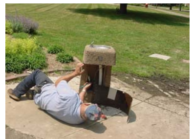
Field Services fixing a water fountain.
