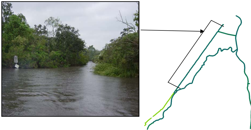
Figure 28: East Bank in the Engineers Canal
