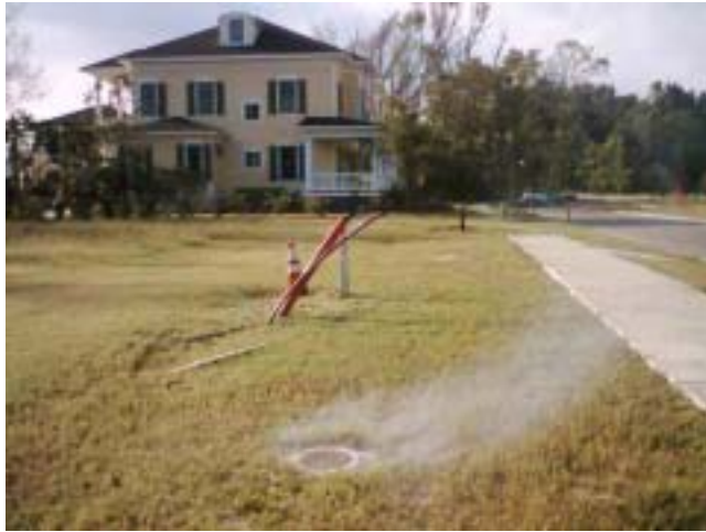
Figure 8. Smoke from a manhole. This photo indicates that either the frame or the manhole seal requires repair. Crews can estimate the time, materials, equipment required to perform the repair, and accessibility.
