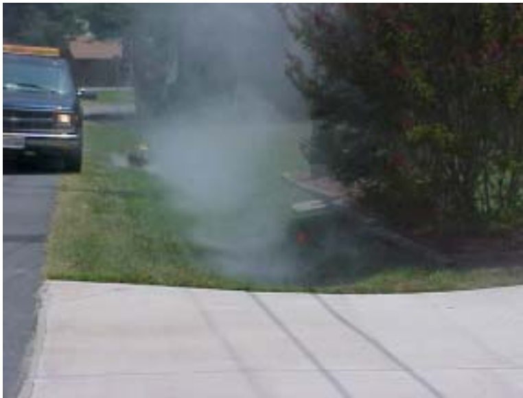
Figure 7. Smoke from a hole in the ground. A picture communicates much more than just tabular attributes. It also indicates the severity of the defect.
