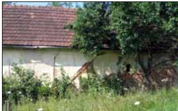
Abb. 6: Damage to a building, caused by active soilcreep
