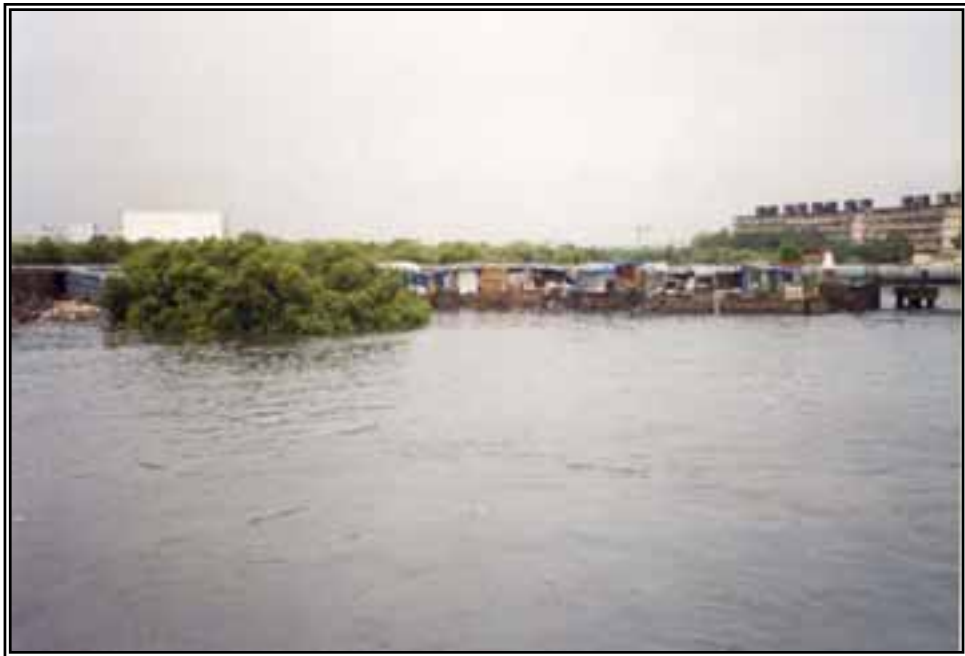
Plate 2: Photograph showing encroachment of slums at Mahim-Bandra creek
