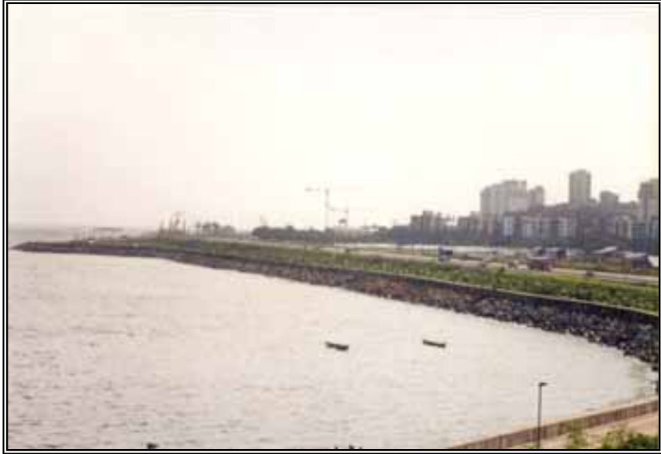
Plate 1: Photograph showing Bandra reclamation
