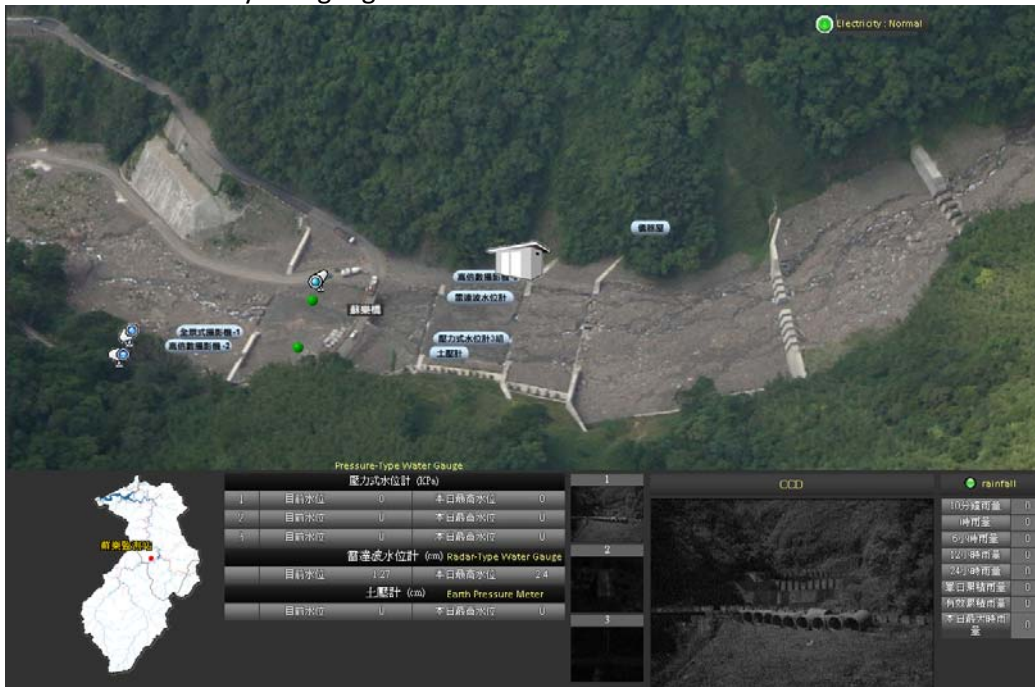
Fig.2 Demonstration platform shows all data from on-site instruments
