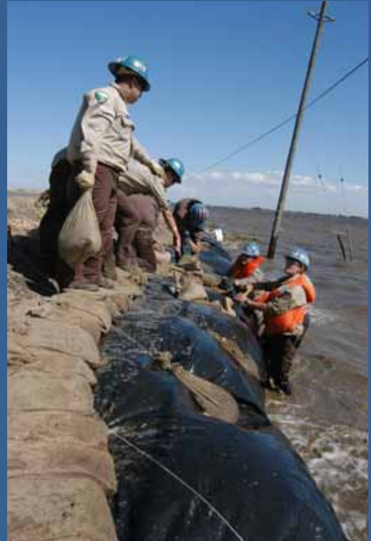
California Conservation Corps Crew Reinforces At-Risk Levee
