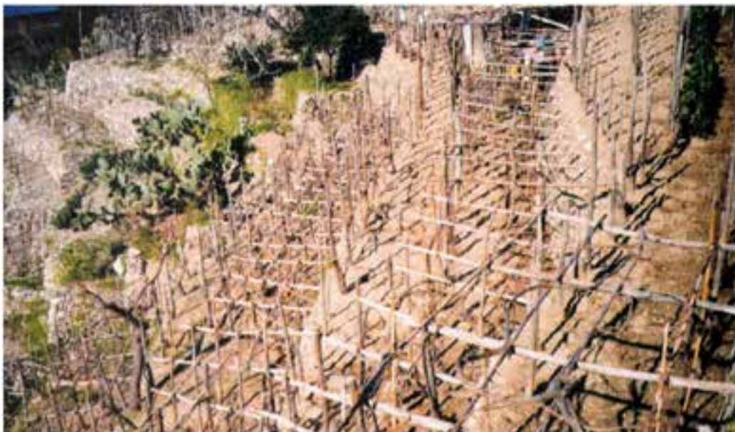
Figure 10. Case study: Landscape Unit “Costa Viola”. Terracing
