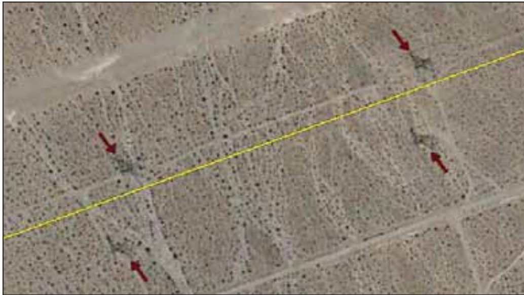
Figure 3.3: Validating Utility Data - The solid yellow line depicts the transmission data used. The red arrows indicate the transmission towers found on California NAIP aerial imagery. In this instance a polyline depicts one corridor housing two transmission lines (2010).
