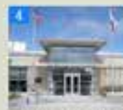
Police and Fire Safety Facility
