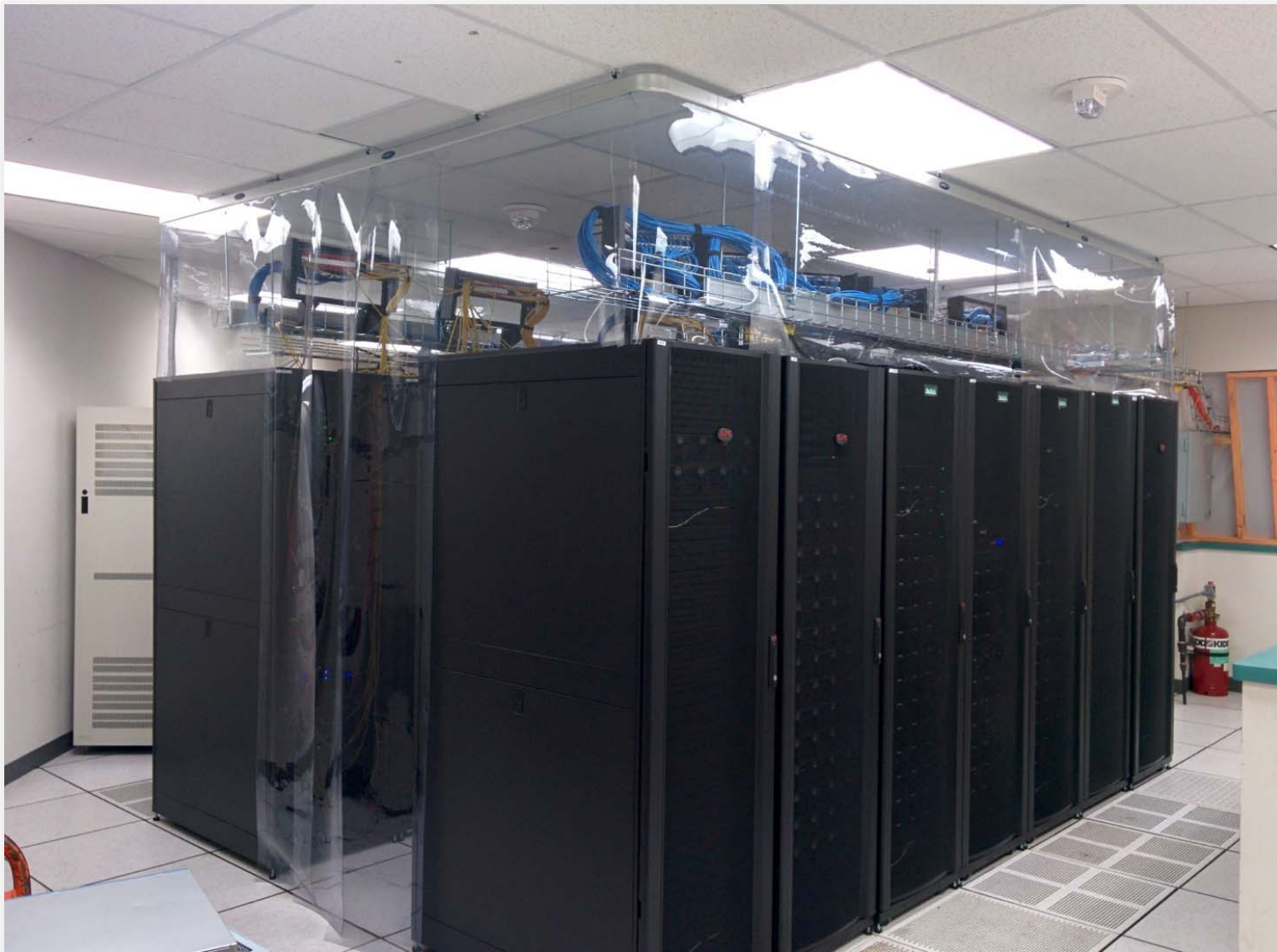
Servers at OIT data center wrapped for cooling
