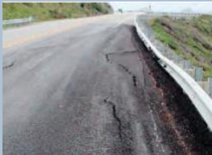
Pavement cracks
