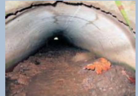
Sediment blockage
