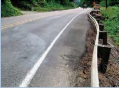
Guardrail settlement
