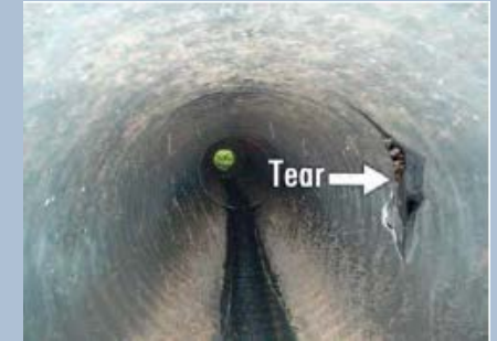
Cracking
