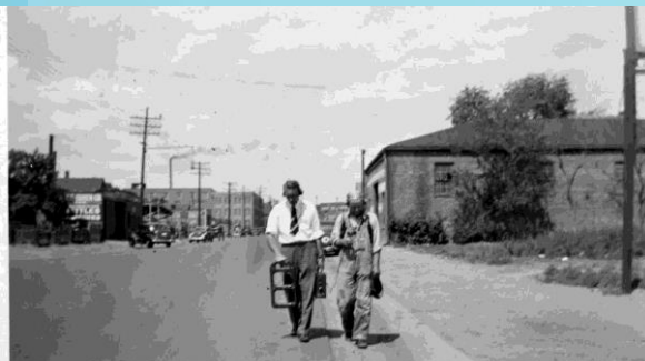
5661 June 13, 1938. Pipe locating device demonstrating on W. Colfax Ave. and 2nd St.
